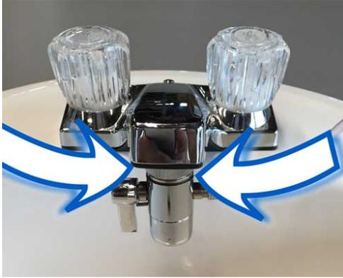
Check to make sure there is a gasket between the diverter valve and the faucet. To do this, turn off your faucet and unscrew the diverter valve.
